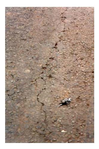
(a) Longitudinal crack in the near-side wheel-path
