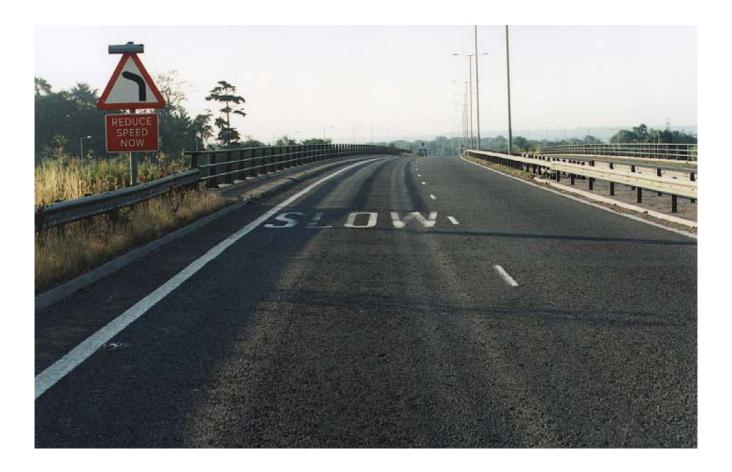
Figure A4 Surface rutting extending onto a bridge deck
